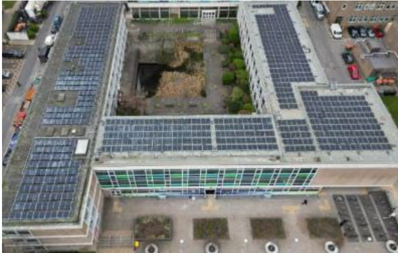
Glyndwr solar array, part of 1800 panel install
